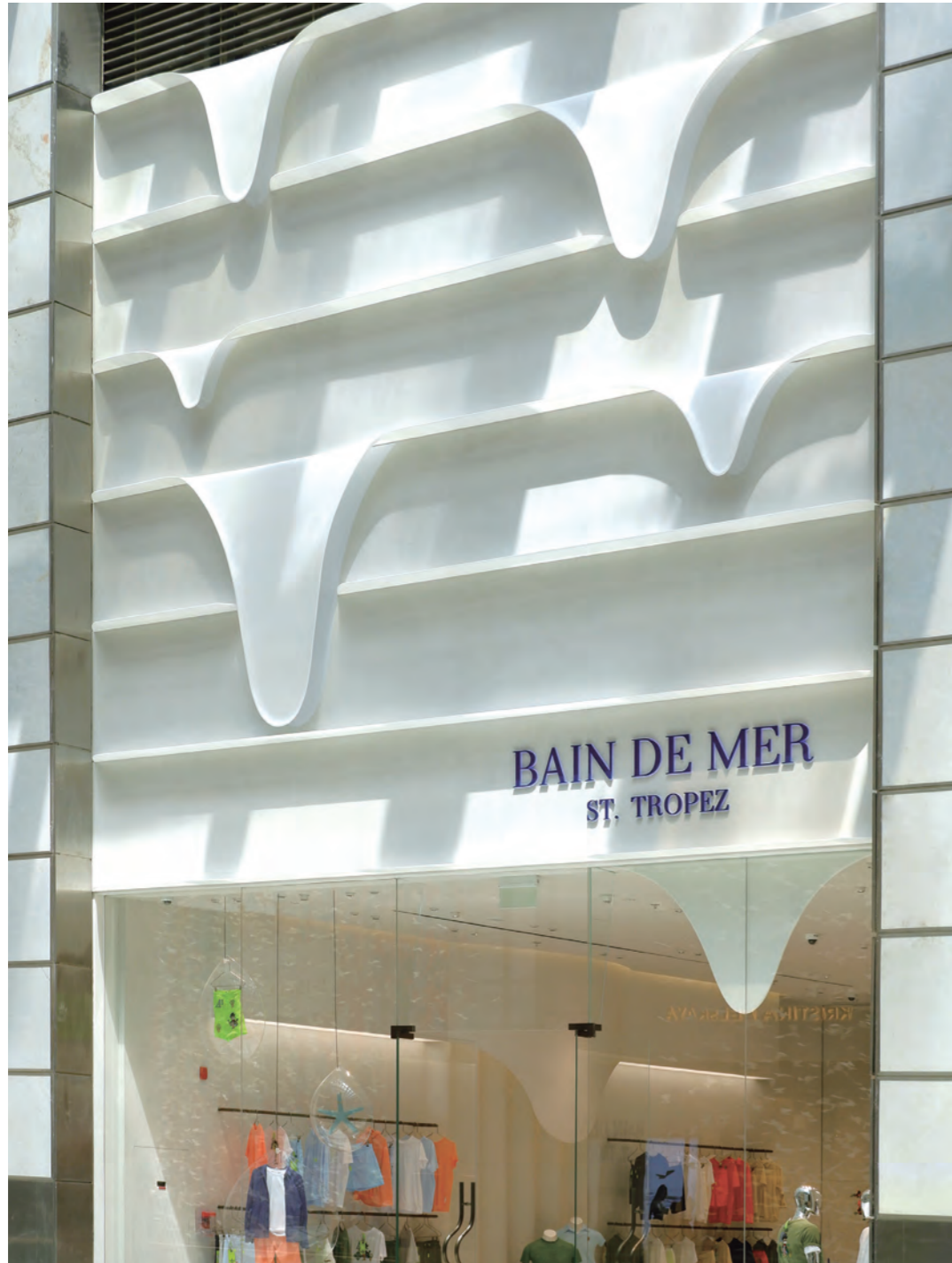
Location : Dubai Material : S028 Alpine White Fabricator : Cube Wooden & Internal Design Accessories Industry LLC.
